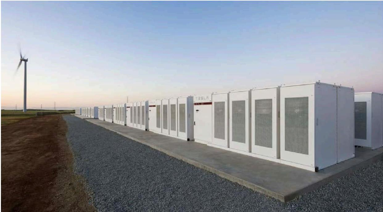
The Hornsdale Power Reserve, a 100-megawatt battery storage facility in South Australia using Tesla lithium batteries.
