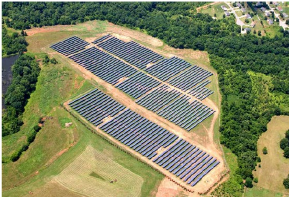
An example of a utility-scale solar facility preserving existing mature vegetation and topography.
