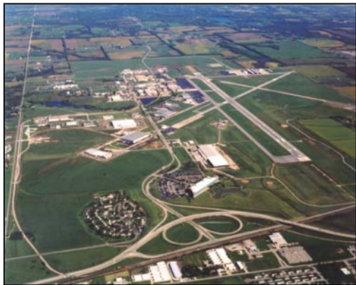
New Century AirCenter looking north-northeast
