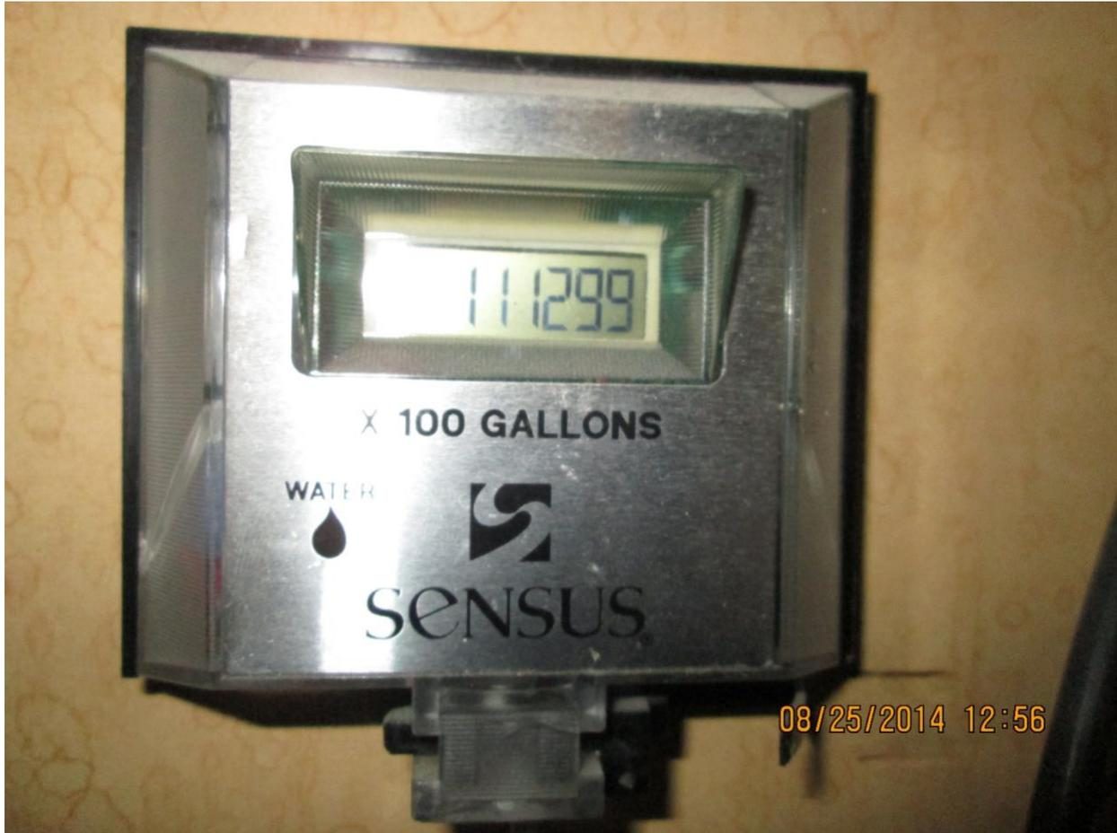
The meter read on this particular dial is recorded the same, by reading from left to right. The information provided clearly states the meter has a multiplier. The multiplier is 100 and is reflected on this meter as X 100 gallons. This would be logged as “11129900”
